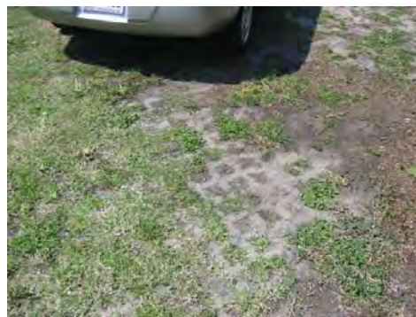
Pulling grass and weeds from the joints can damage parking surface if roots are firmly established in the bedding layer.
