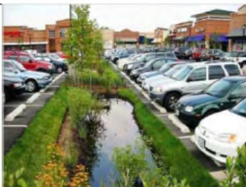
Grass filter strip: accepts sheet flow from the parking lot
