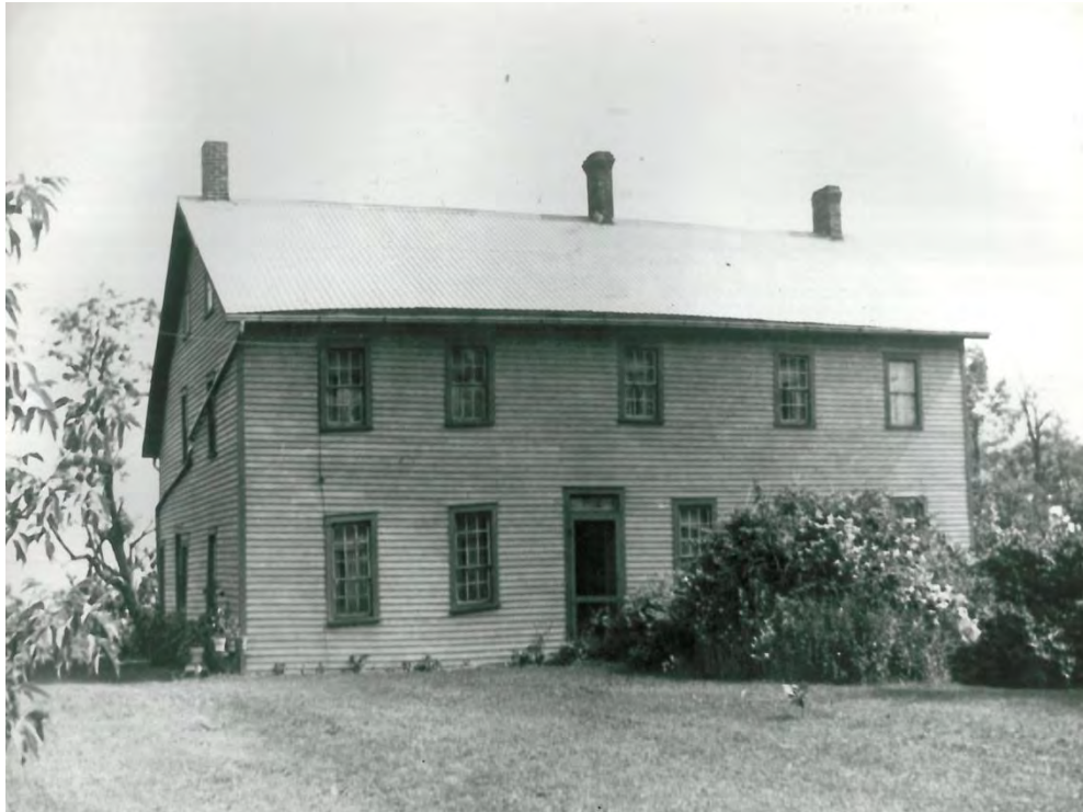
Plate 11: The Hoover Frame House, circa. Late Nineteenth Century, built around the Hoover log cabin which was located on the left side of the house as seen in this photograph
