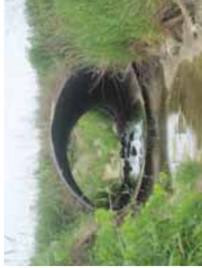
Photograph 2. Perched culvert
