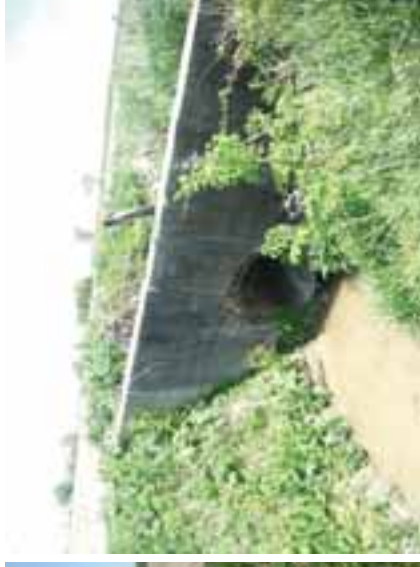
Photograph 3. Perched culvert
