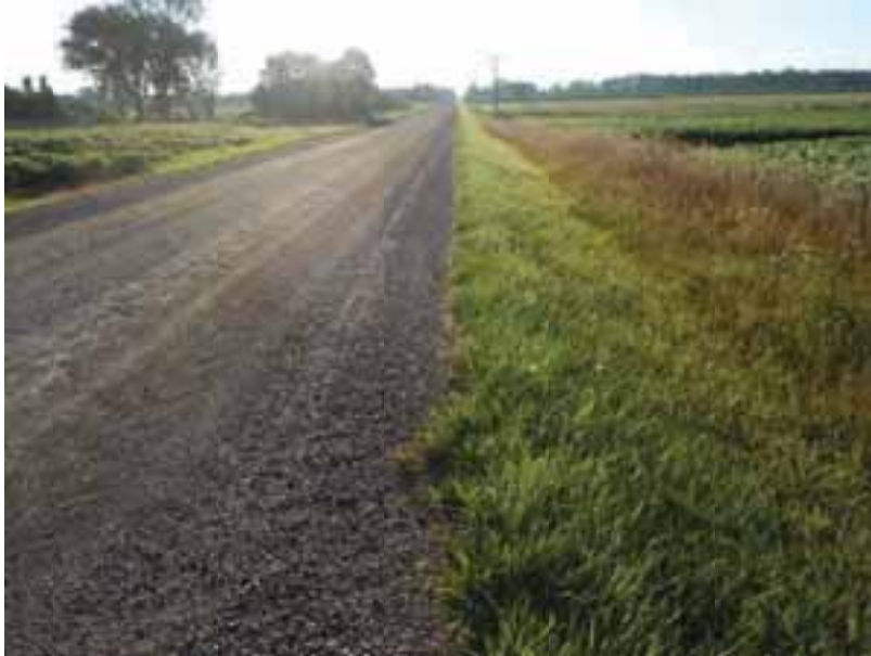
Photo 88: Disturbed ROW – JER1040, facing east
