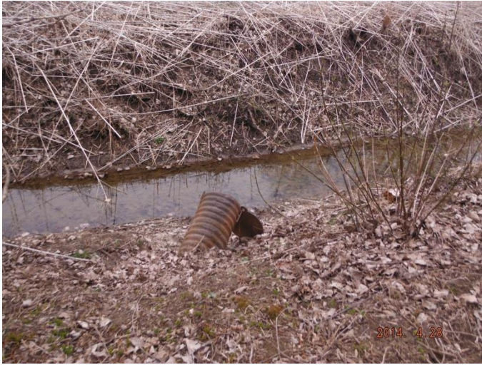
Photograph 5. ↑ Location of culvert draining out into watercourse east of pond.
