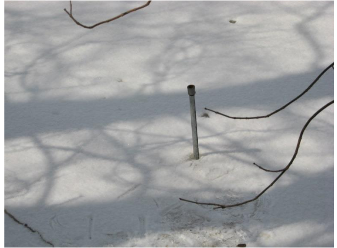
Photograph 6. ↑ Mini-piezometer and staff gauge installed at east end of pond, facing west. Note staff gauge is buried beneath ice.
