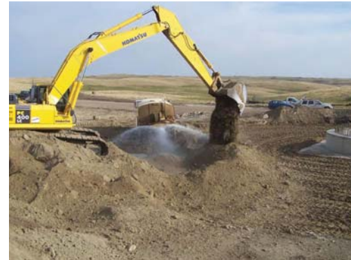
Construction equipment moves soil as part of the site preparation process.
