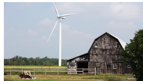
(NextEra's Summerhaven Wind Energy Centre)
