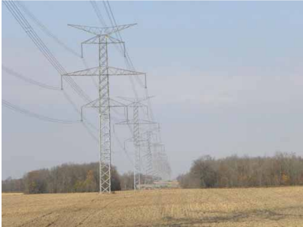
Plate 1: Transmission line, looking north from the intersection of Staffa Road and Tower Line.
