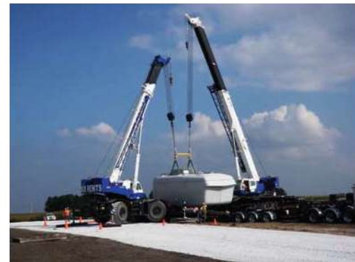
A wind turbine component, known as a nacelle, is lifted from a truck.
