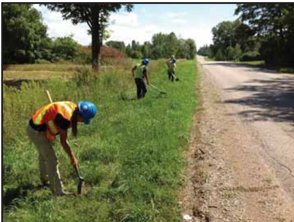
Image 28: View of Crewmembers Test Pitting to Confirm Disturbance at BLW1065 (Photo Taken August 7, 2013; Facing South)
