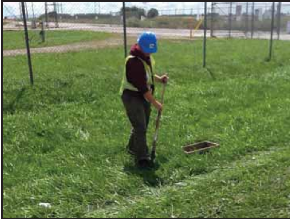
Image 51: View of Crewmembers Test Pitting to Confirm Disturbance at BLW1129 (Photo Taken August 15, 2013; Facing South)
