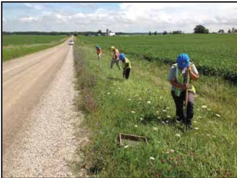
Image 40: View of Crewmembers Test Pitting to Confirm Disturbance at BLW1088 (Photo Taken August 8, 2013; Facing East)
