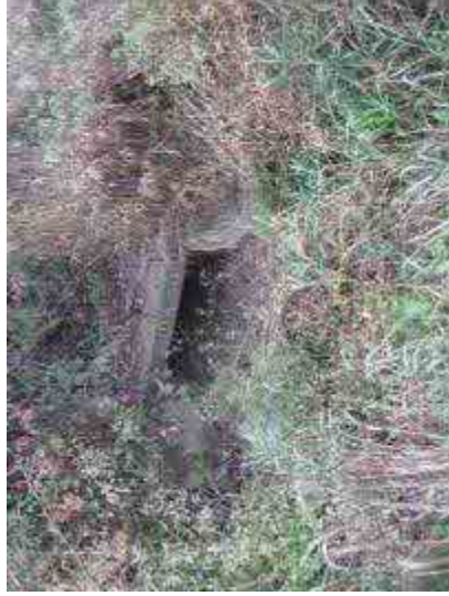
Photograph 1. View of cement culvert ↑
