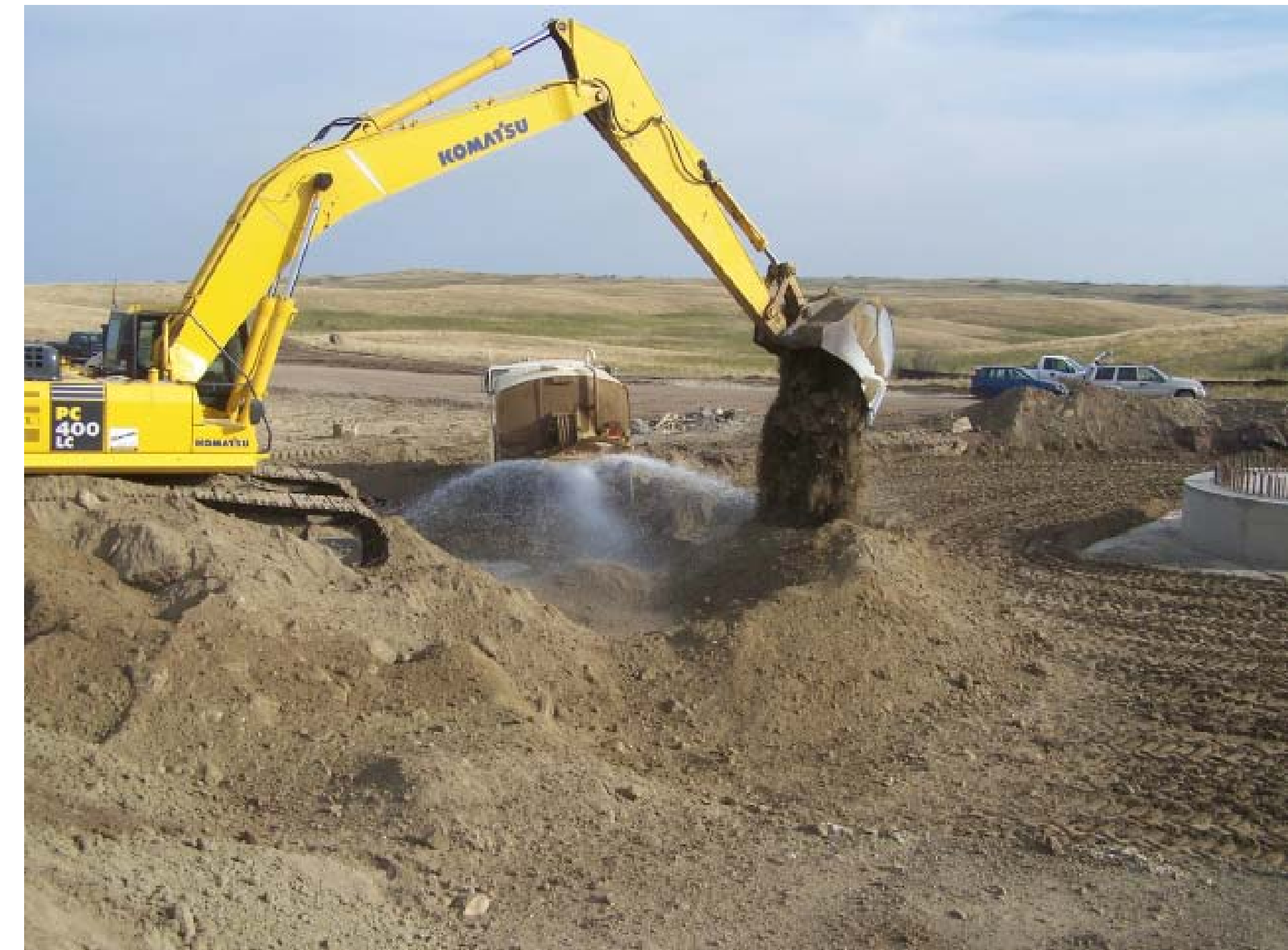
Construction equipment moves soil to backfill a turbine foundation.
