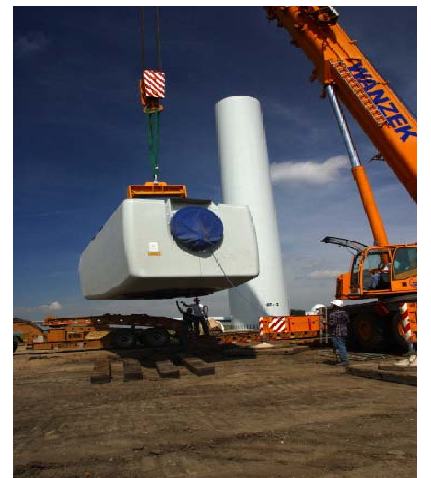
A wind turbine component, known as a nacelle, is lifted by a crane
