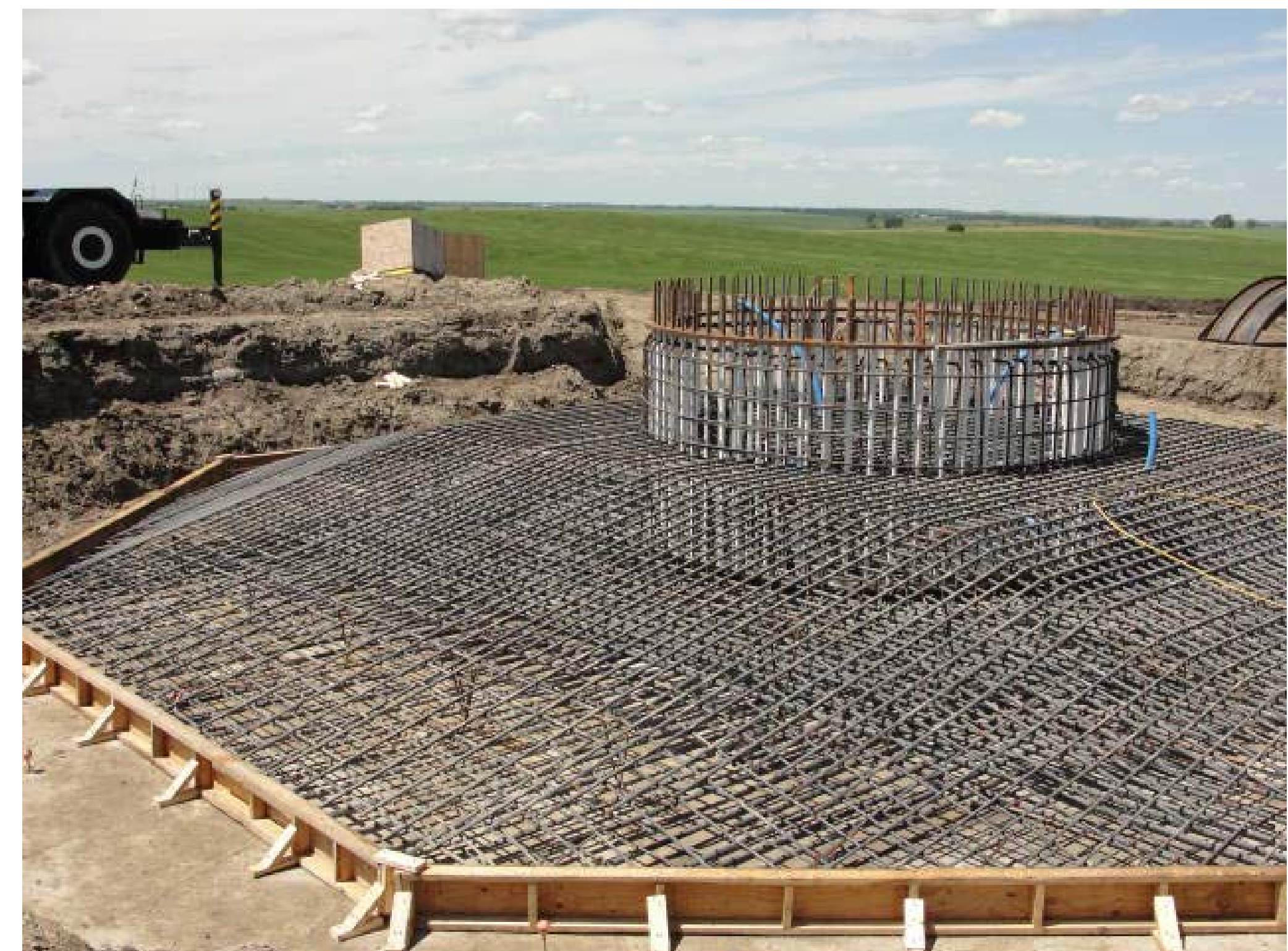
Turbine foundation is framed for concrete pour.
