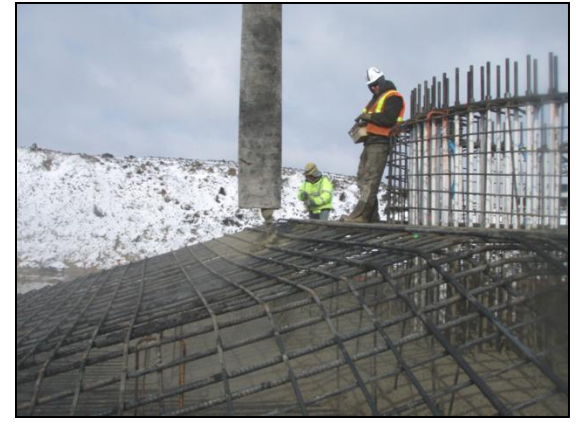
Prepare turbine foundations
