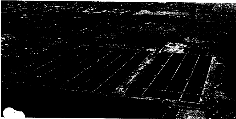
(Images of Sarnia Ontario Solar Farm)
